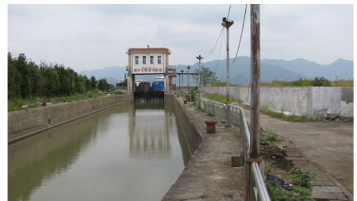
2 ↑ The dam of Changtang Reservoir
